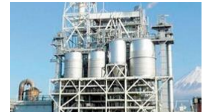
Environmental Facilities & Plants
